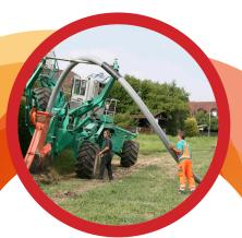
**Ploughing in** – a form of narrow trenching, which ploughs a trench of the exact size for the pipe and feeds the pipe directly from a coil into the trench. The process is fast, but only works in soft-dig areas with mainly stone-free soil.
