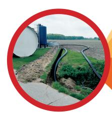
Open trench – this is the most common technique. Narrow trenching can be used if the installer can work safely to make any joints. Damage to the jacket pipe from poor handling can be repaired using a suitable repair set available from the manufacturer.
